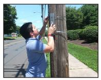
IMPORTANT: The area of the Black Cat Radar Recorder that you are aiming toward the road is the picture of the Black Cat, as shown in the picture here. The radar head adjusts up and down to allow you to find the best angle.
