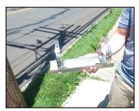
**Step #2** - For the most accurate results, the bracket should be installed so the Black Cat Radar Recorder is facing traffic on a 45 degree angle. Once you have determined this position, wrap the bands around the pole and place the bracket.
