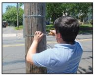
**Step #4** - Insert the pegs on the back of the Black Cat Radar Recorder's mounting bracket into the large holes of the pole mounting bracket and slide the Black Cat Radar Recorder down to secure it in place.
