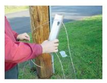
**Step #2** - For the most accurate results, the bracket should be installed so the Radar Recorder is facing traffic on a 45 degree angle. Once you have determined this position, place the bracket.
