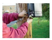
**Step #6** - Once the Radar Recorder has been setup using the *Collect* software (refer to the next chapter), close the lid and lock it.
